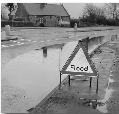
Above: Blocked drain flooding beside the garage.
