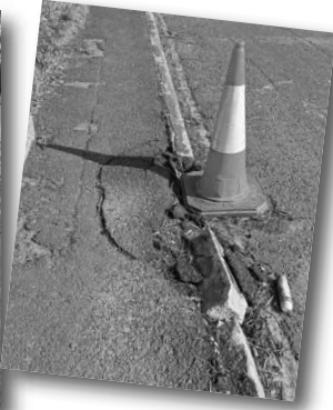
Above right: Damaged kerb, Hexham Road.
