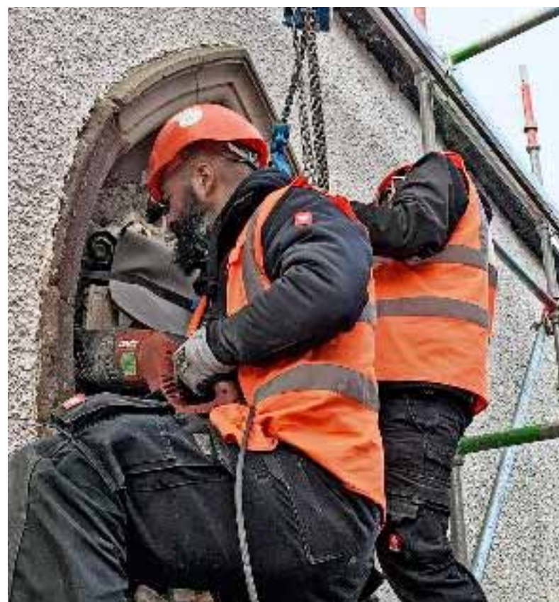
Conservation Workers start removing decorative stonework from library wall
