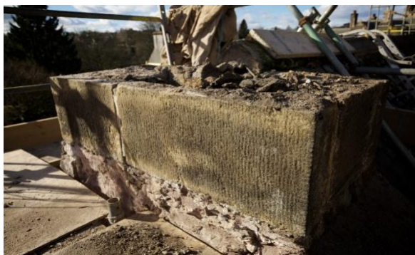
South chimney: Picture Tom Astbury
