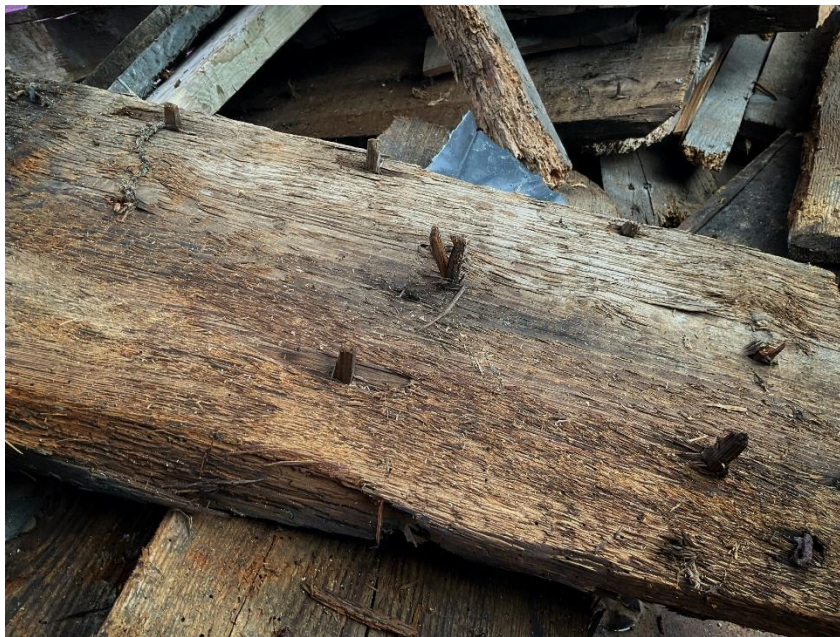
Wooden pegs on old timbers
