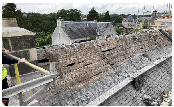
**The east elevation**. Some of the boards have timber pegs visible from inside the attic space. The roof boards are in very poor condition, soft and worm eaten and not suitable for fixing slates. Replacement timbers will match the original dimensions. Staggered joints will make the roof structure stronger.
