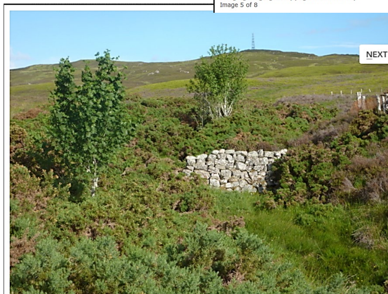
This is the remains of the dam at Monbuie drove stance where cattle would have been able to take a well earned drink. Copyright: Neil Ramsay
