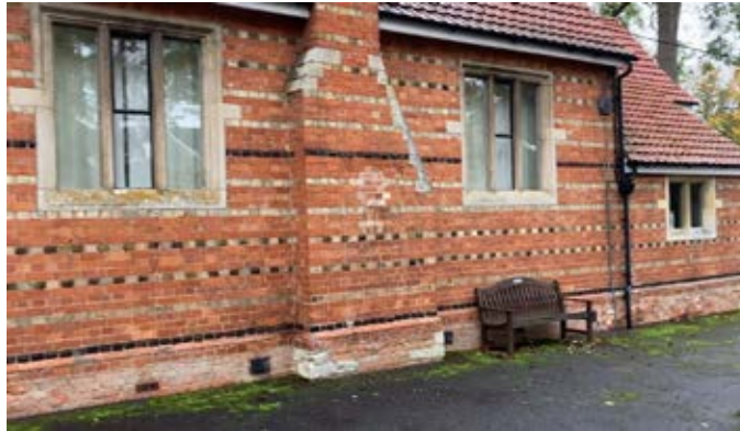
Figure 7: The distinctive patterned brick of the village hall.
