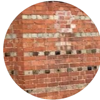
RED BRICK WALL WITH DETAILING
