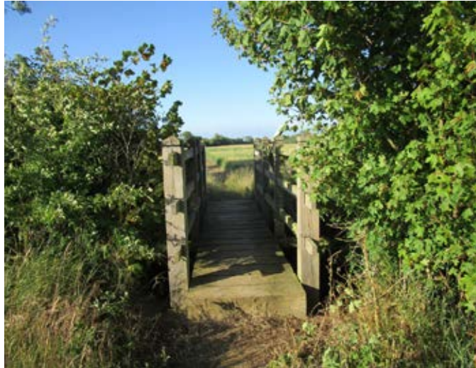
Figure 38: Footpath bridge to the north east of the village.
