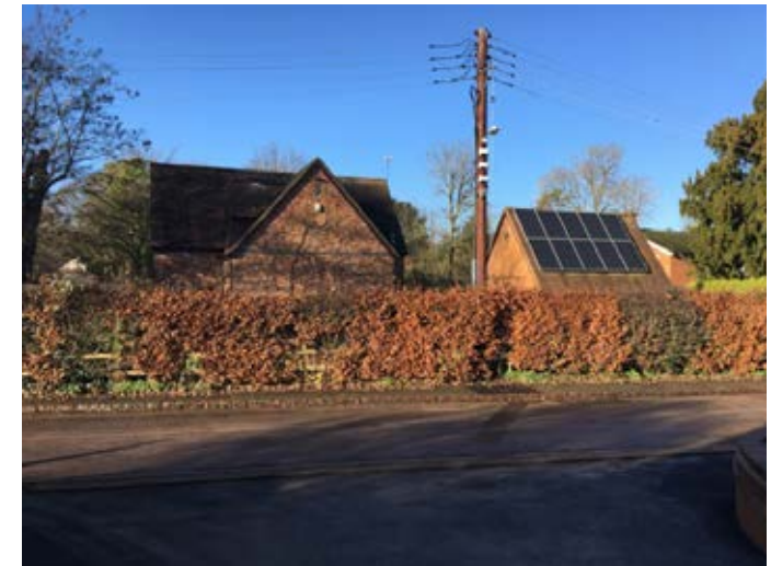
Figure 57: Example of solar panels on a garage roof in Hargrave.
