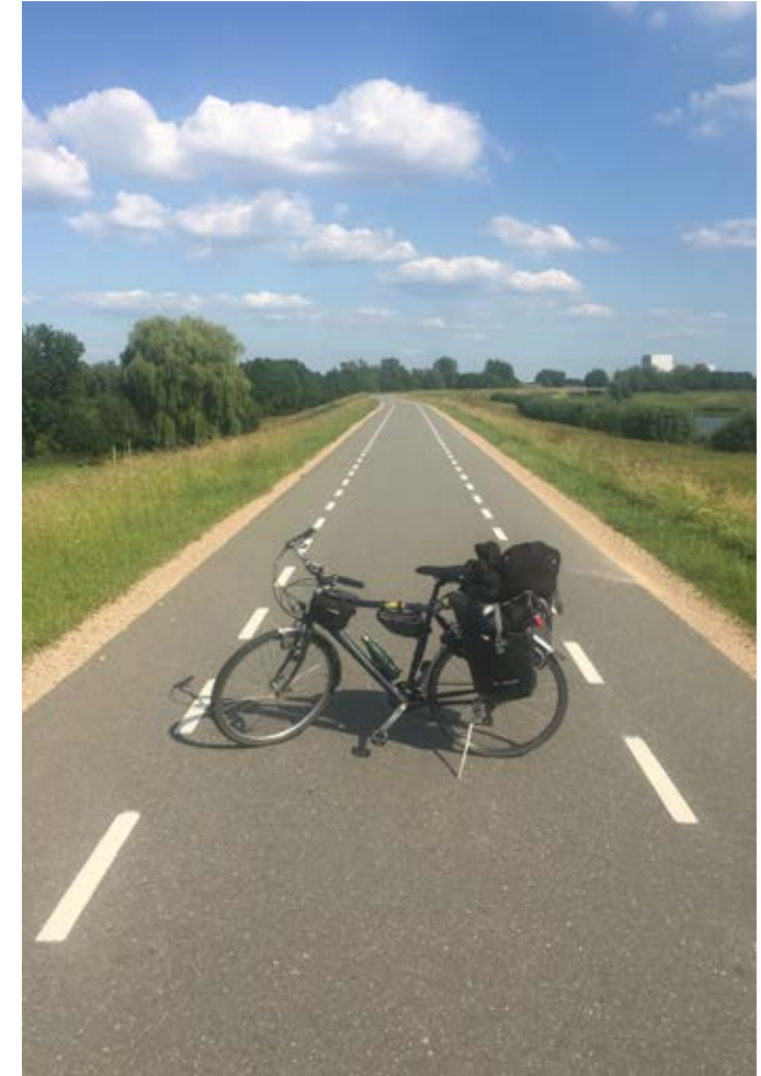
Figure 37: Simple white line pedestrian and cycle lane markings, leaving a single lane for traffic.
