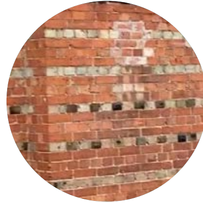
RED BRICK WALL WITH DETAILING
