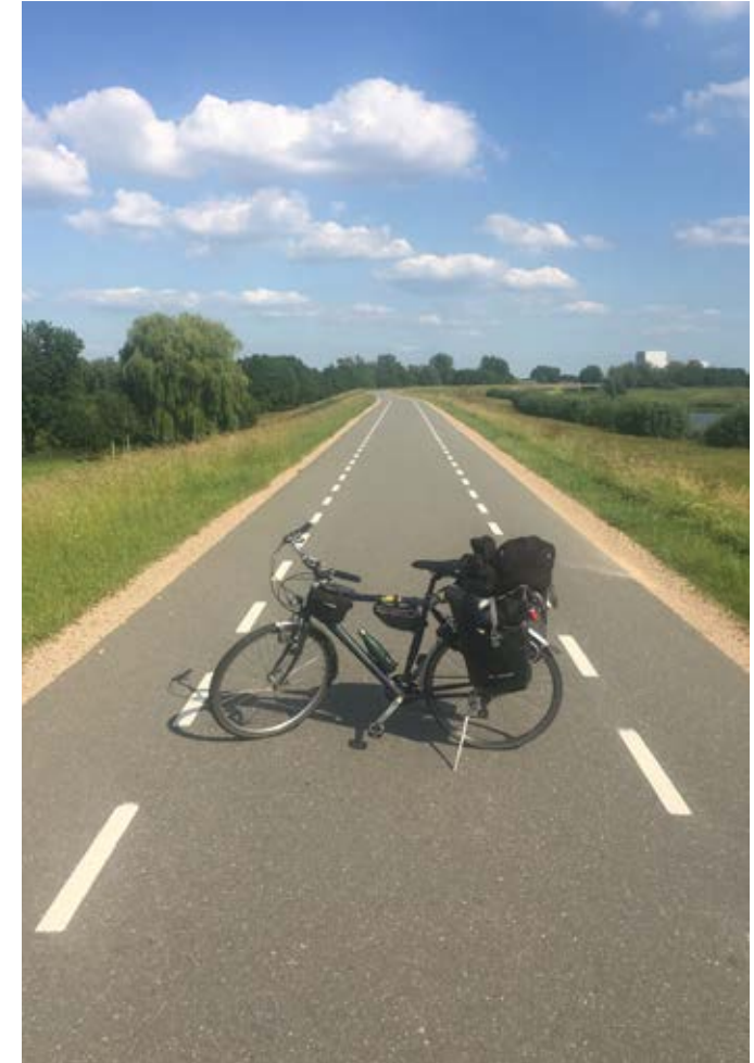
Figure 37: Simple white line pedestrian and cycle lane markings, leaving a single lane for traffic.
