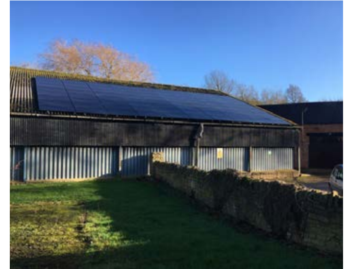
Figure 55: Solar panels on barn in Hargrave.
