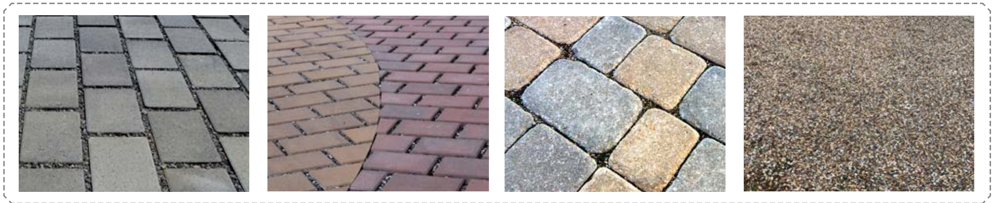
Figure 61: Examples of permeable paving.
