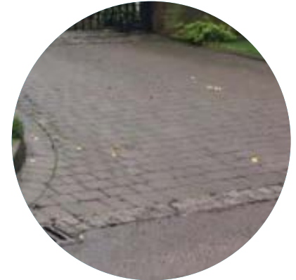
BRICK PATTERN SLABS AS POROUS SURFACE MATERIAL
