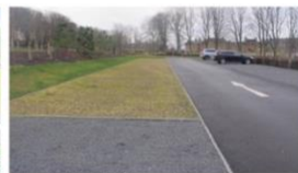
Plastic paving with gravel infill foreground
