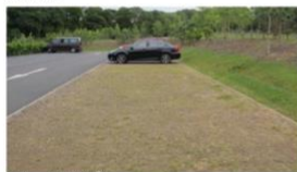
Plastic paving infilled with gravel
