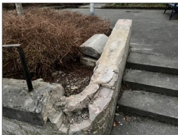
Repeated damage to the coping on the Fleshmarket Steps Photo: Grant Kinghorn
