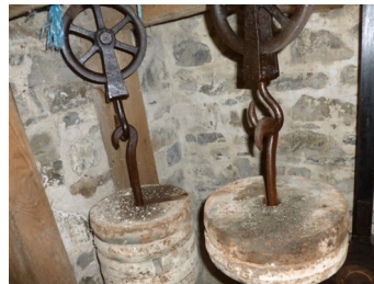
Repeater that is used to synchronise the clock faces
