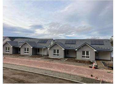
The housing project is nearing its completion. The site offices have been taken down, the block paving is nearly finished, turf is being laid in the eight gardens and the fences are being erected.
