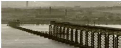
Collapsed Navigational Span
