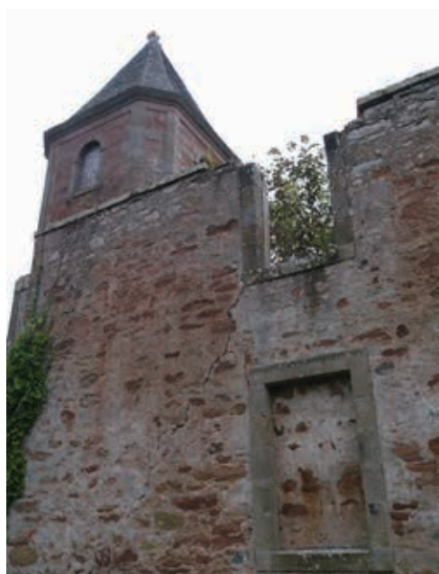
The clearly seen long crack in the west-facing wall presents the serious danger of a collapse.
