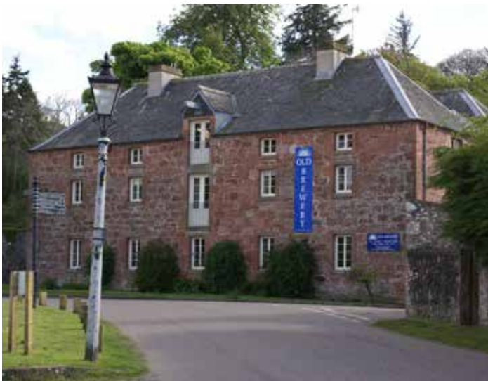
The Old Brewery in Cromarty dates from about 1785, and was restored to its present use for educational courses and workshops in 1989. The building has been Category B listed since 1971.
