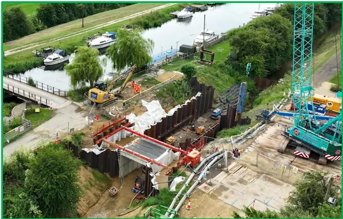
Figure 1 - Aerial View of Construction Site
