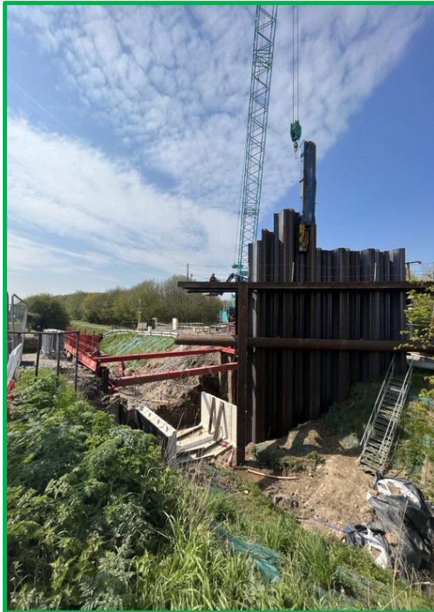
Figure 2 – Installation of sheet piles – upstream of the new culvert
