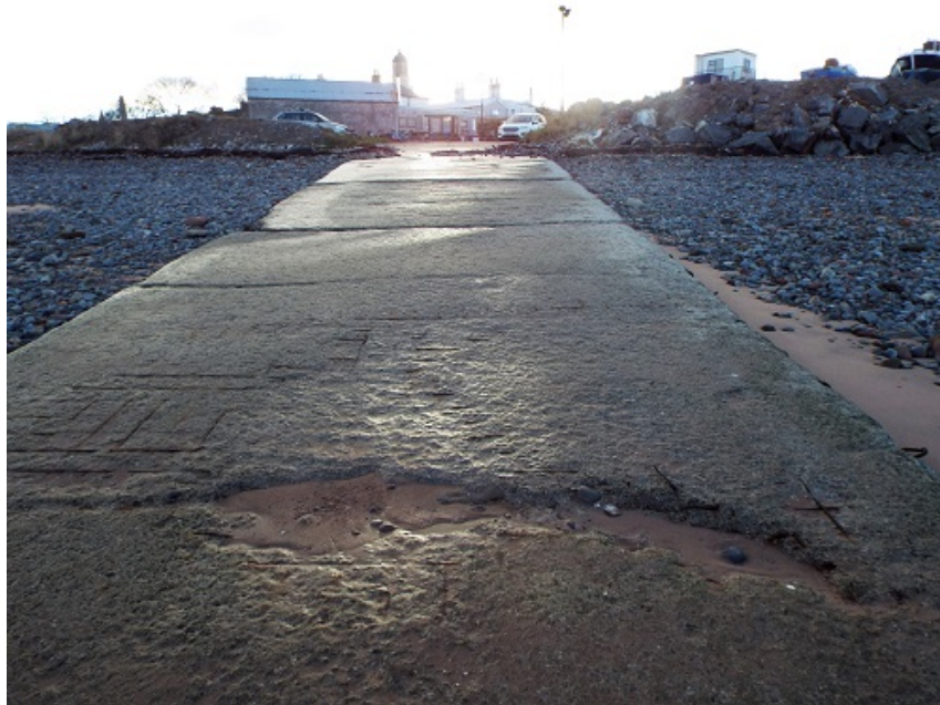
Image: The ferry slipway on the Cromarty side.
