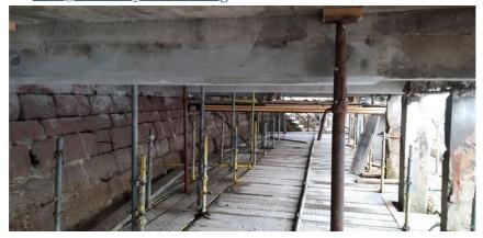
This photograph illustrates the condition of the soffits, columns and beams which require to be repaired or replaced prior to the new fenders being installed. Also work in progress which includes hand-finishing in places.
