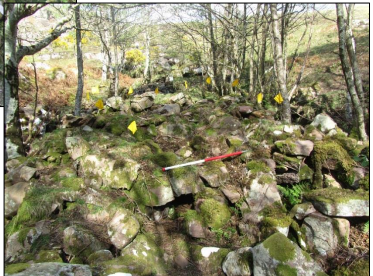
Figure 12 (right): The north part of Building 16 with the edge of the bowl highlighted by flags. The void with lintel stones can be clearly seen
