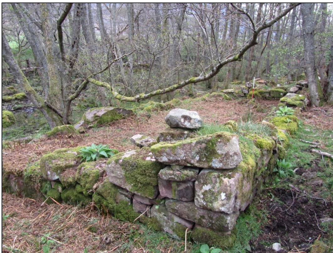
Figure 2: Building 18 looking west
