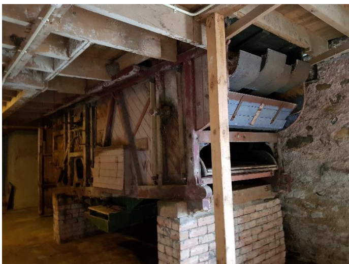
Figure 18: The threshing machine supported on brick plinths
