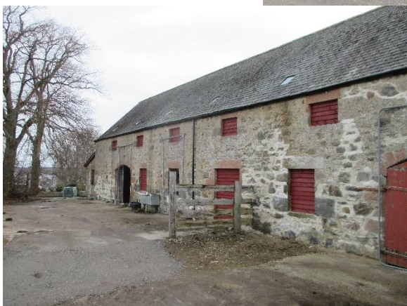
Figure 15: The rear NW aspect Note the doorways into the lower floor of the north wing. The upper windows, now boarded, represent the upper floor of N wing, with windows in the sloping roof. © Anne MacInnes
