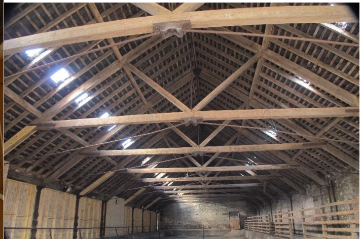
Figure 25: The roof of the cattle court. Note, in the 1878 newspaper article each couple was estimated to weigh "a ton and a half".
