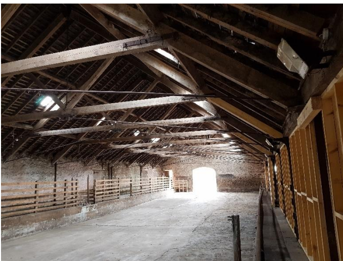
Figure 24: The western cattle court, looking S Note the raised passageway on the left to allow access along the length of the court.
