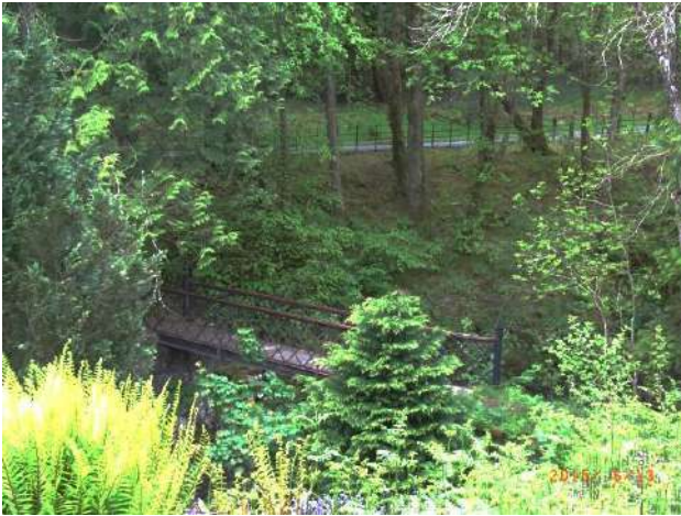
Wrought iron bridge
