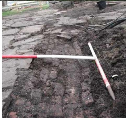
The central row of bricks forming the drainage channel were laid flat. On either side, four rows were set on their sides, rising at a shallow angle. Here the inside three brick rows have been removed when a shed was built in the 1970s. The gutter ends in a sump against the far wall, which was not
