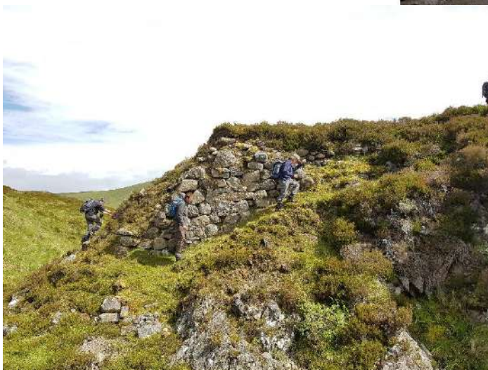
Exploring the Bridge abutment near Aultguish Inn
