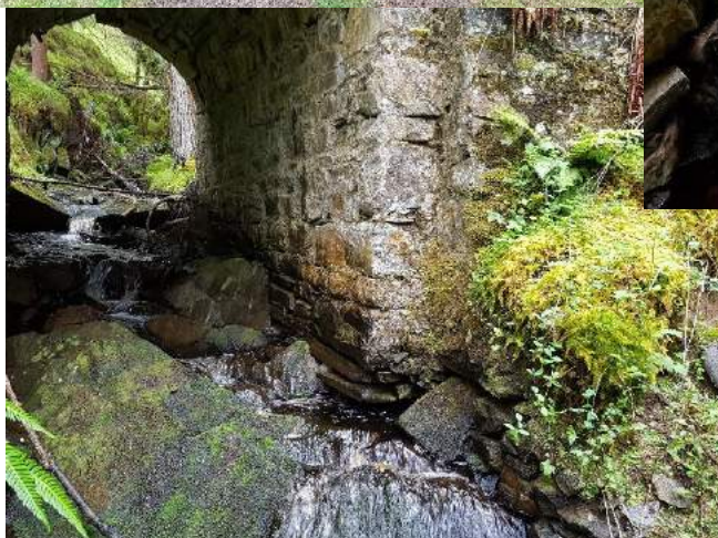
FN60 Eroding NE foundations of bridge 08.07.16 © Roland Spencer-Jones
