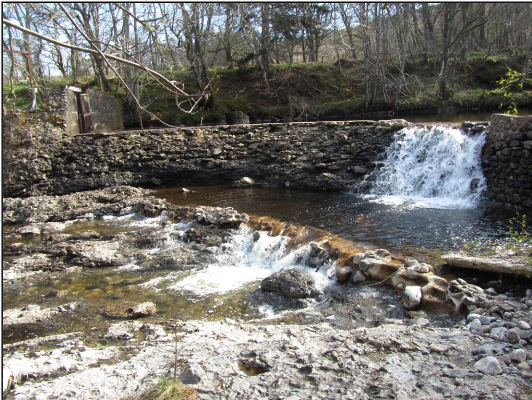
The dam, viewed from the north, with the remains of the earlier dam in the foreground
