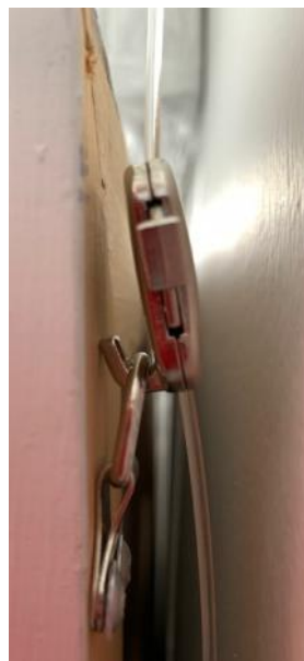
Right: how a hanging wire/hook works
