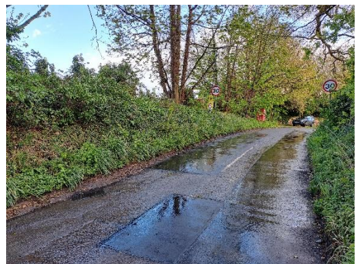
Road surface into the village
