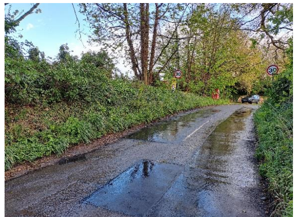
Road surface into the village
