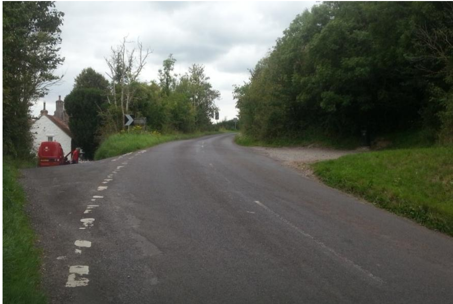
WR/Rackley Lane Junction. Looking in a westerly direction. Rackley Lane on left of photo, blind bend in centre and entrance to/exit from PROW AX15/6 on right
