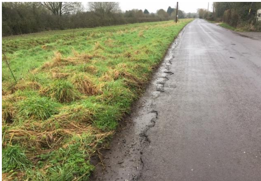
Long straight section of OCR. Photograph also shows verge damage caused by HGV's, Tractors and trailers.
