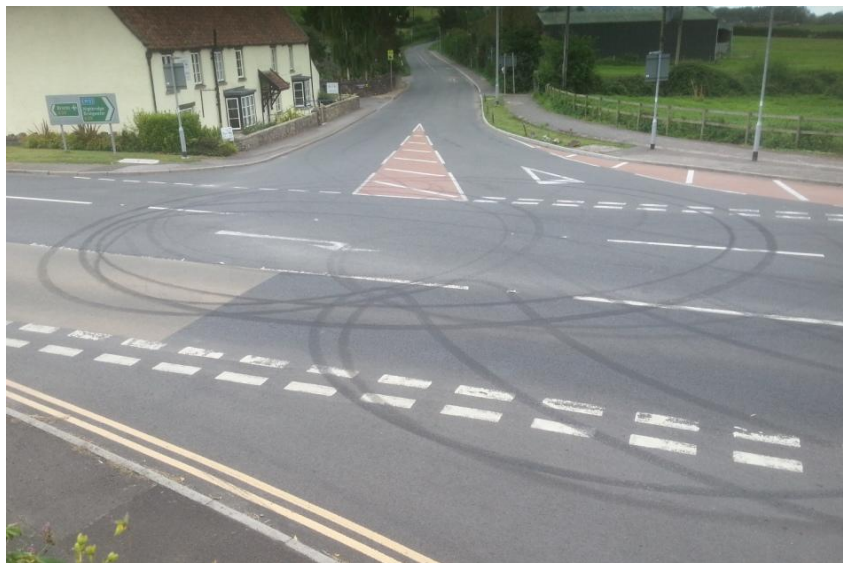
Tyre skid marks at New Inn following 'donut' incidents shown in video
