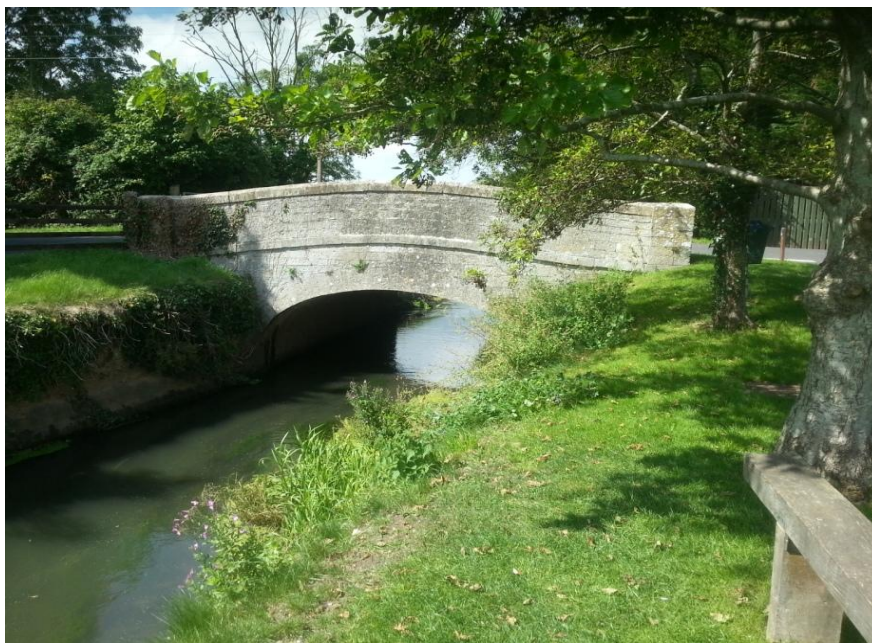
Bow Bridge over the Axe Yeo
