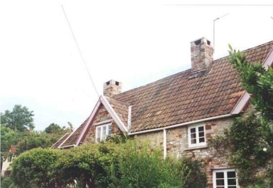
Originally roofing would have been thatch probably and single Roman, replaced by slate for the 'up-market' house and pan-tiles for others.
