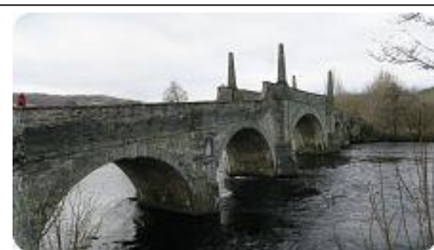
Wades Bridge at Aberfeldy
