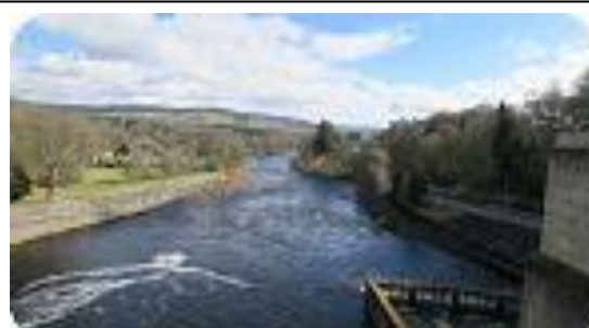
Pitlochry Fish Pass, Hydro Dam
