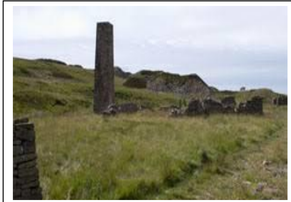
The Musburry Heights Quarry Chimney
