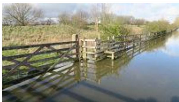
The flooded stile and footpath adjacent to the A59 Clitheroe
