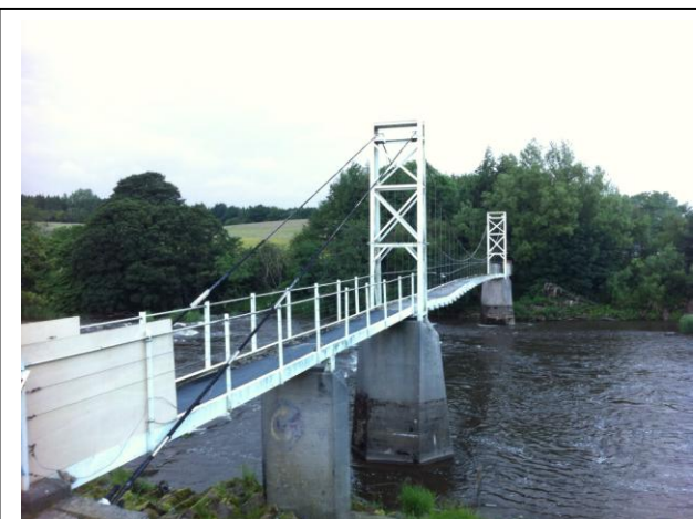
The new footbridge at Dinkley
