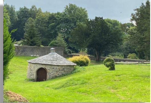
The Well House at Bolton Hall
