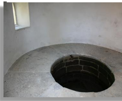
Inside the Well House
