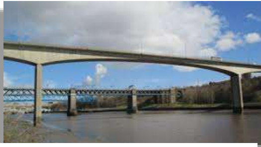
The Tyne Bridge at Redheugh
