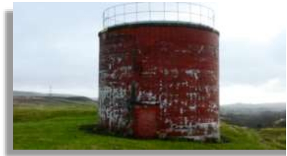
Sough Tunnel Air Vent
