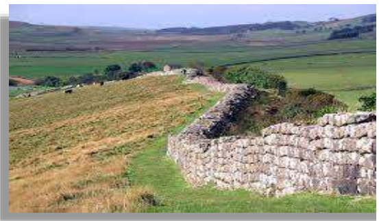
A Section of Hadrian's Wall
