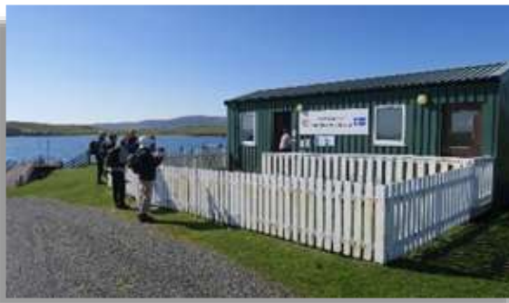
Ferry terminal waiting room
