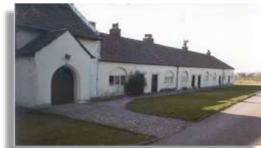
Alms houses attached to Lathom Chapel, Lathom Park, Lathom
