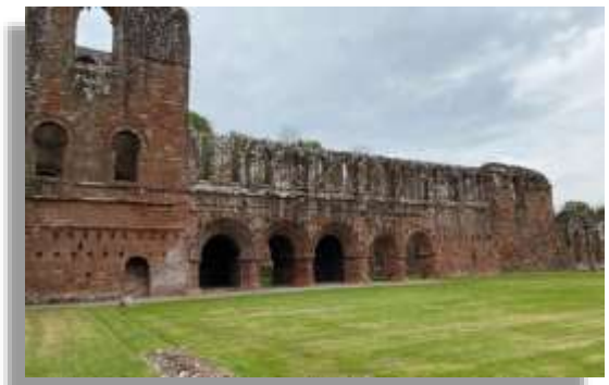
The Cloisters from the west tower
