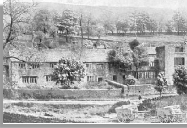
Wycoller Hall as it would have looked in Charlotte Brontë's day.
