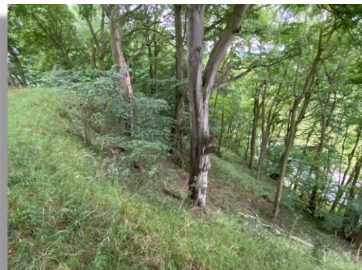
The collapsed side of the motte at Castle Haugh Eleanor
