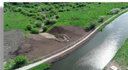
The work completed 1st June 2022
