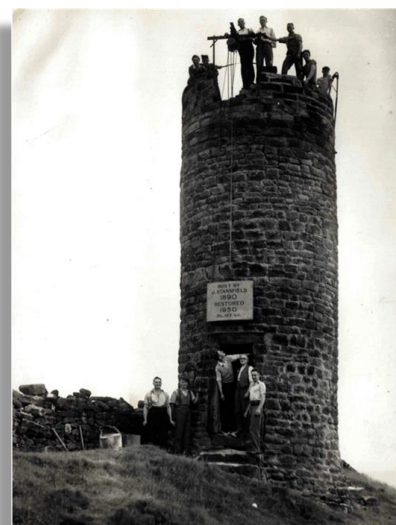
Repairs to the Blacko Tower
