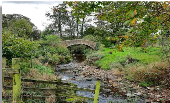
Fairy Bridge at Bashall Eaves
