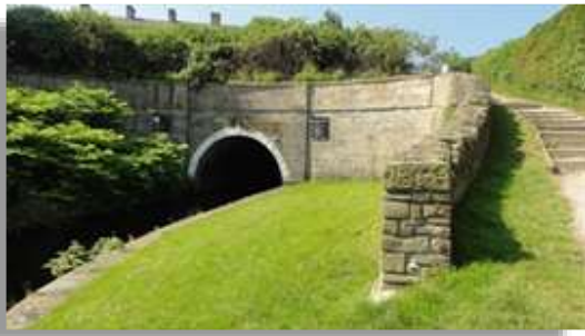
Gannow Tunnel on the Leeds Liverpool Canal
