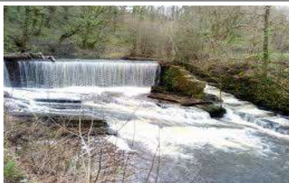
The Weir and Fish Pass on the River Yarrow
