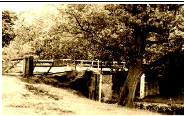
The bridge over the Leeds Liverpool canal at the Sun Paper Mill Feniscowles
