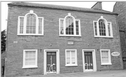
The former Glasite Meeting House in Perth High St.
