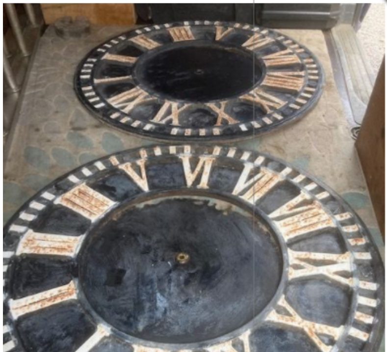
The clock face on the way to being repaired
