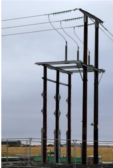
Figure 2.3 Typical Cable Sealing End Compound
