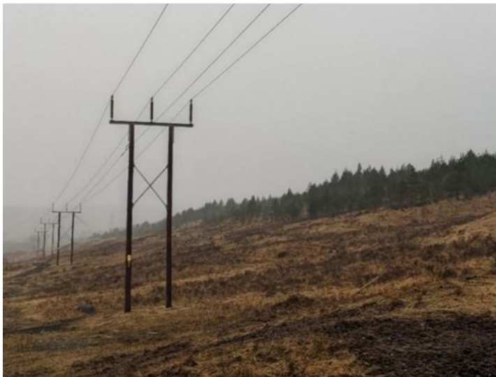
Figure 2.2 Trident 'H' Wood Pole Example
