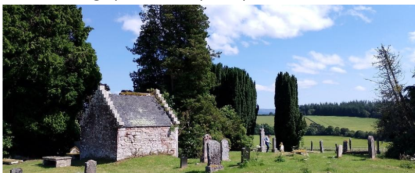
Figure 2. St Duthac's Church ruins and graveyard at Easter Suddie. The building is a family vault conversion, adjoining the ruins
