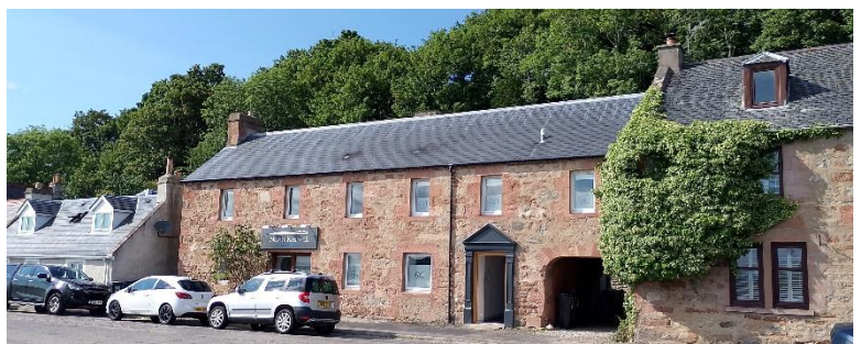
Figure 7. The former North Kessock Mission Hall
