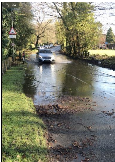
Current flooding south of the Gole Road site across School Lane at Causeway Bridge when flash floods occur
